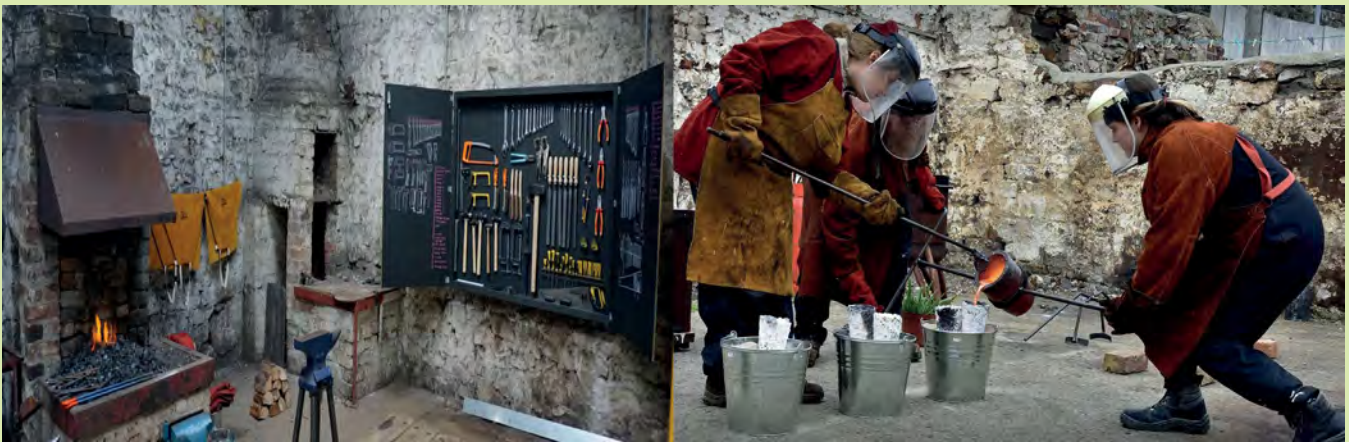
As part of the STAMP project, at the historic and derelict site Cei Llechi (Slate Quay) in Caernarfon, the old forge was reinstated to create a temporary community forge and focal point for testing and discussing future uses of the site.
